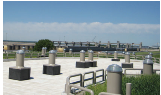
A 5,000 sq' observation deck overlooks the Mississippi River, Melvin Price Locks and Dam, and Clark Bridge.
